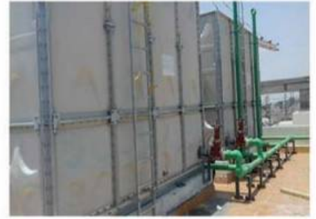
COMMERCIAL RESIDENTIAL BUILDING-MECCA
